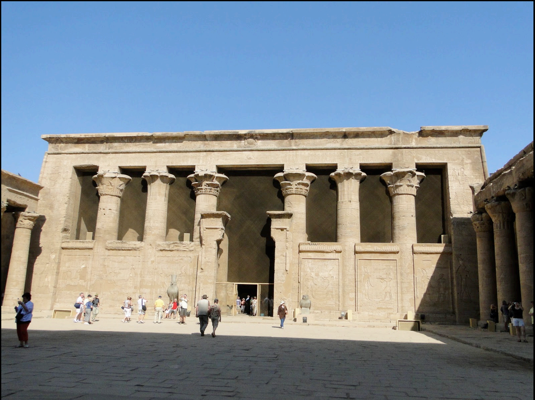
Inter-columnar screen wall between the courtyard and first hypostyle hall, Edfu
