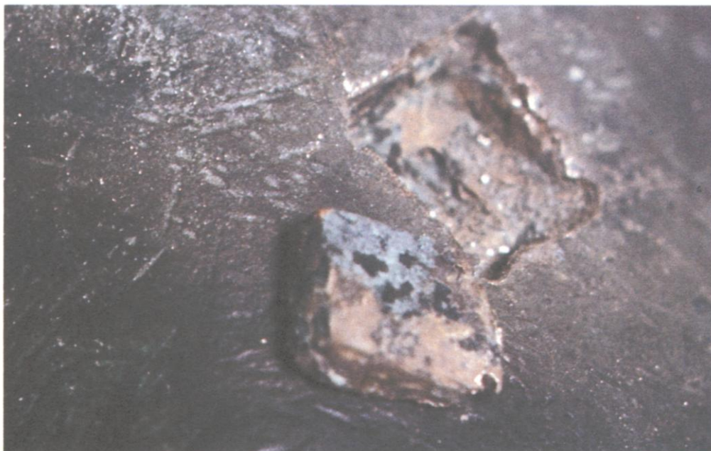
FIG. 13. Underside of repair plug after removal from left rear leg.
